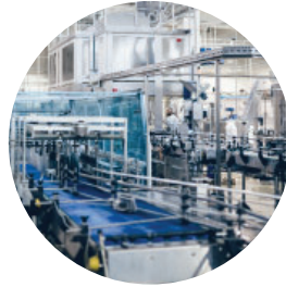
Industrial Water Systems
